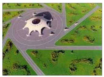
The central dome of this airport contains terminals, maintenance facilities, service centers, and hotels. The runways are arranged in a radial configuration, which allows airplanes to easily take off into the prevailing winds and to avoid dangerous crosswind landings.
