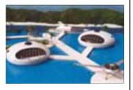
Homes are prefabricated from a new type of pre-stressed reinforced concrete with a flexible ceramic external coating; they are relatively maintenance-free, fireproof, and impervious to weather. Their thin shell construction is mass-produced in a matter of hours. With this type of construction, there is minimal damage from earthquakes and hurricanes.
